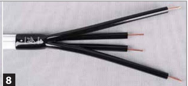
8. Strip the PVC to expose the bare wire.
